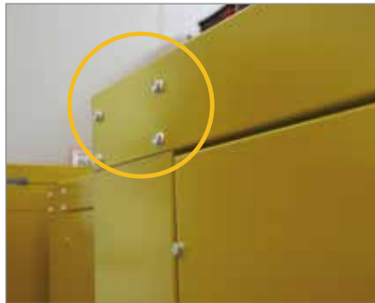
▲ Galvanized bolts Boulons galvanisés
